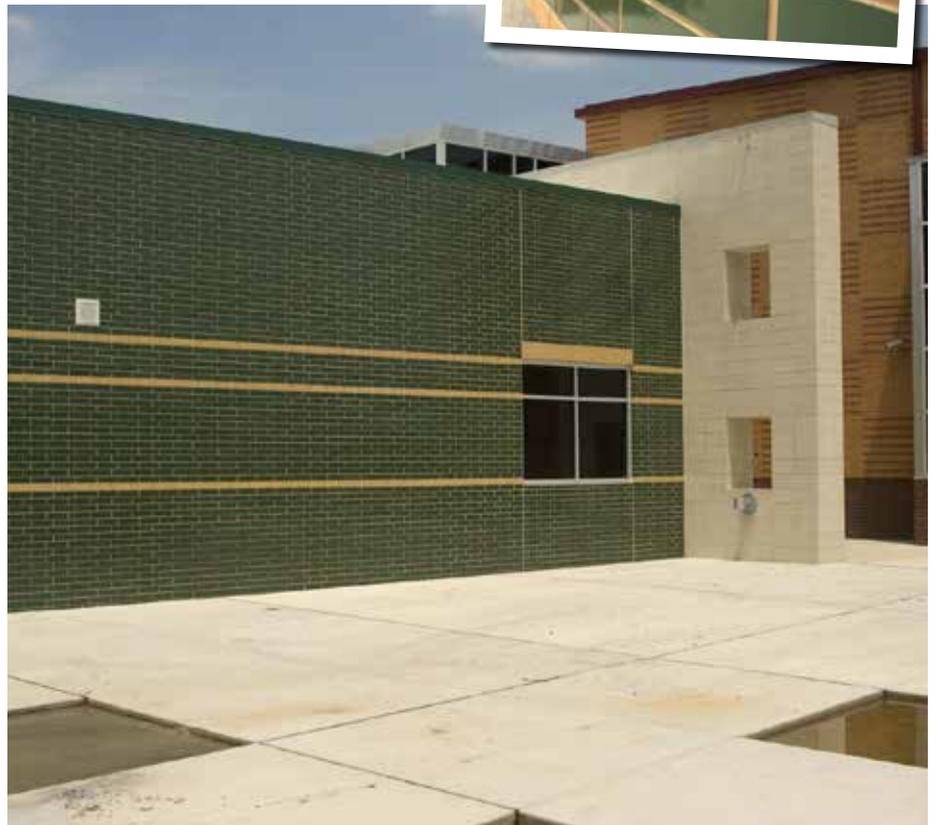
*Ceramic glazed masonry will multi-task in a project's performance, acting as structure, enclosure, aesthetic finishing, acoustic insulation, thermal mass, fire barrier, and partition as in this Walnut Bend Elementary School project.*
